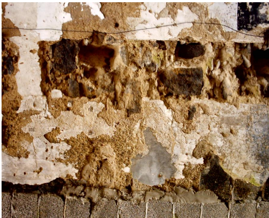
Figure 2 – Extraction of mortars in S. Miguel, Azores
