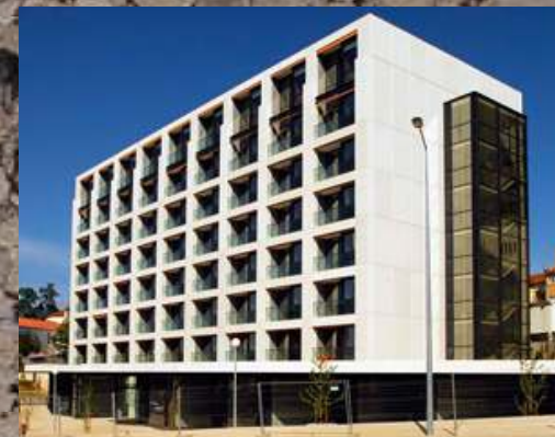
Studio Residence - Coimbra
